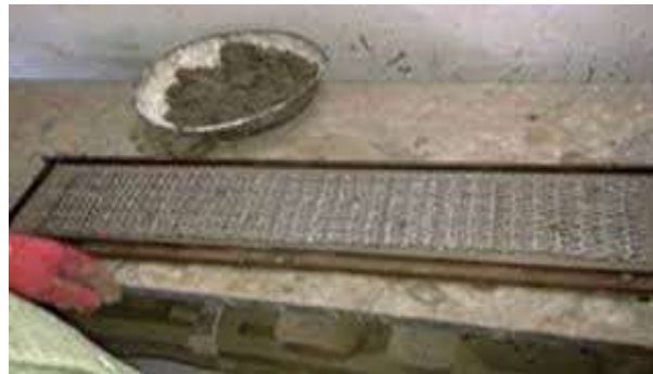
Figur -2 Casting of Ferrocement Panels.
